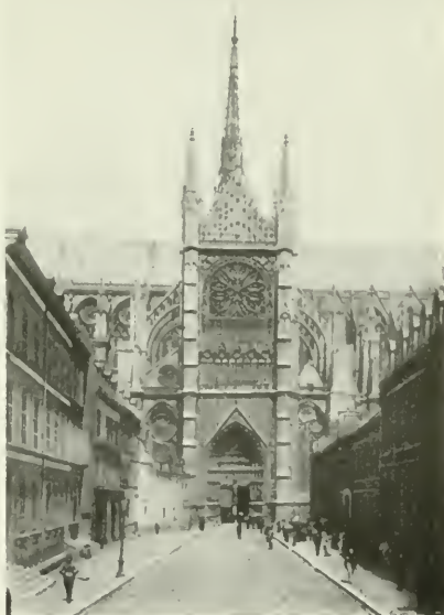
GABLE OF SOUTH TRANSEPT
